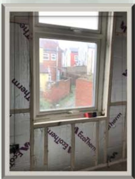
Wall insulation being installed
